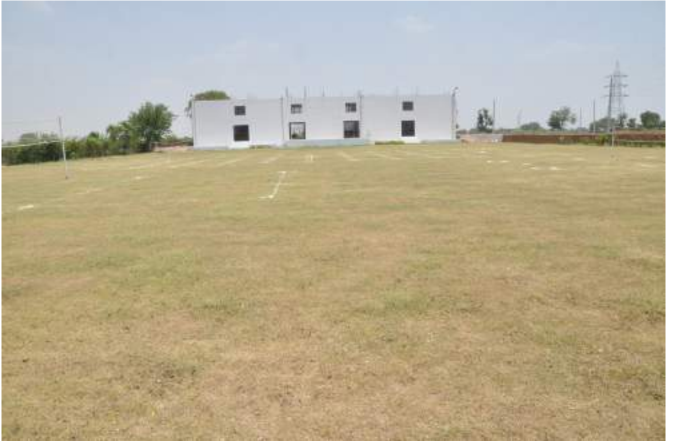
Rear view of the building
